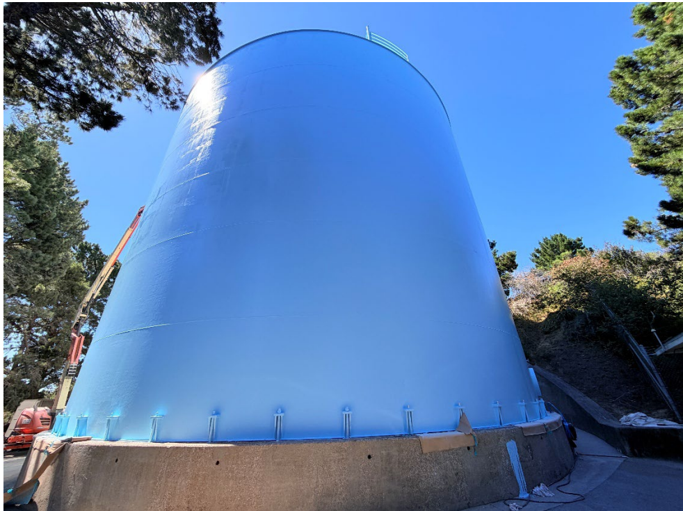
West Belmont (N) – Final coat
