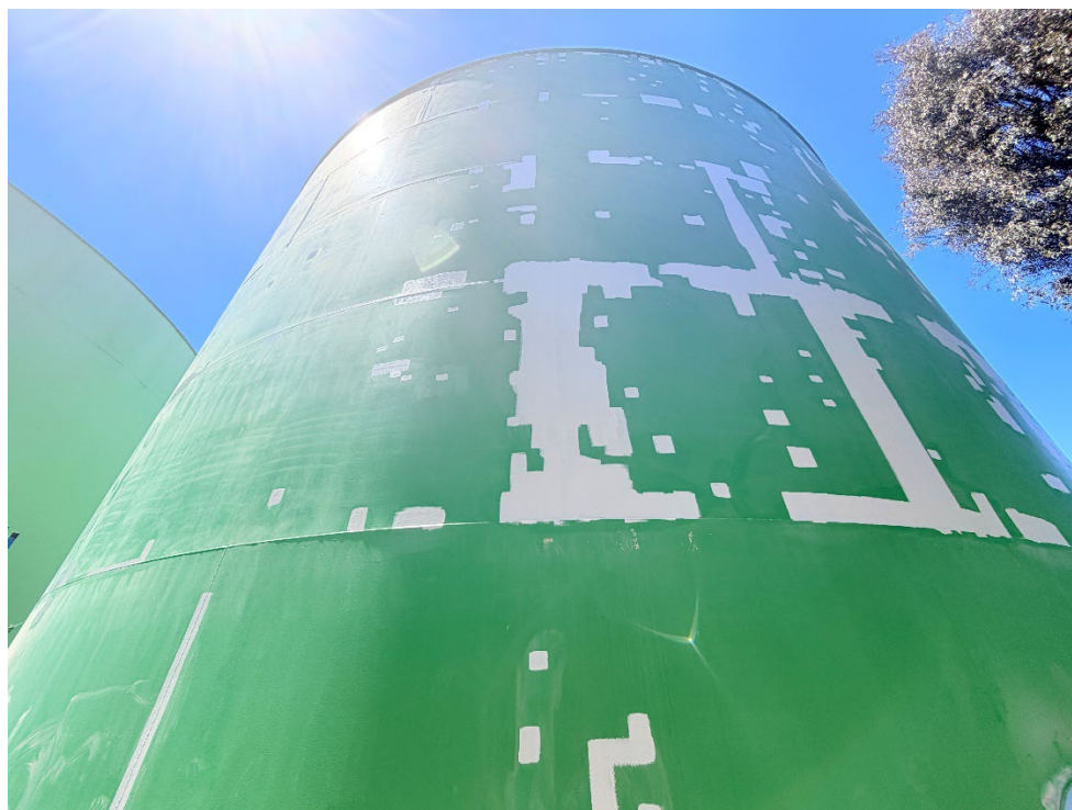
Exbourne (W) – Exterior spot repair
